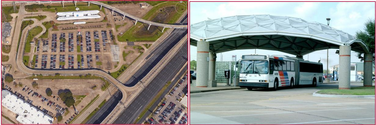
Figure 3-11: - HOV Lane Direct Connector Lanes to Transit Center Bus Only Facilities
